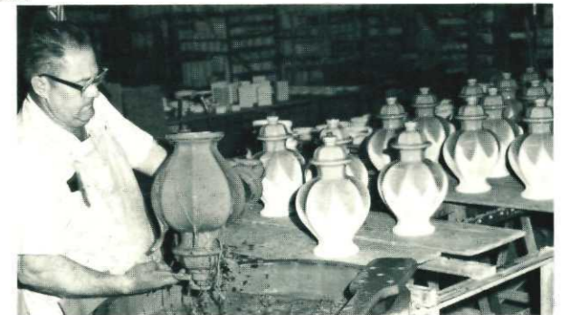
Highly developed glazes are applied by hand to each piece to assure fine quality.
